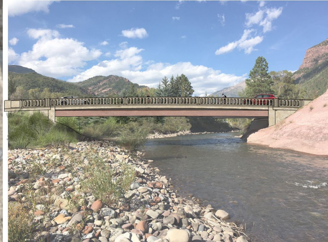
Proposed new bridge with free span of the Crystal and colored girders based on community feedback
