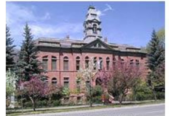
PITKIN COUNTY COURTHOUSE
