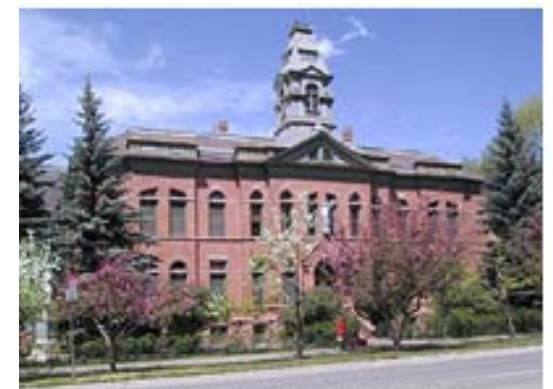
PITKIN COUNTY COURTHOUSE
