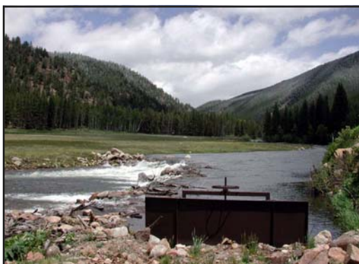
Diversion Structure on Crystal Creek
