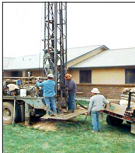
Well construction near Northglenn
